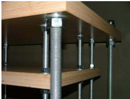
Various stages of construction.
