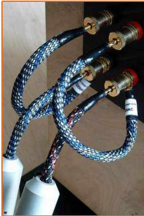
Photo's of the rear with the bi-wiring terminals connected for single-wiring. The cables are by Dyrholm Design Audio from Denmark.
